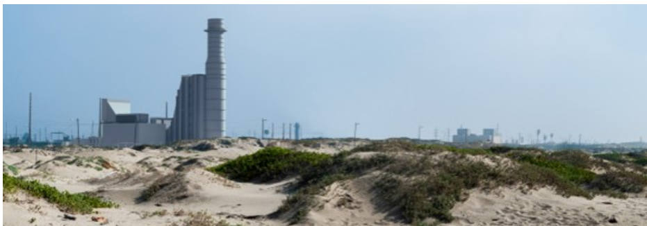
Puente Power plant | California Energy Commission
